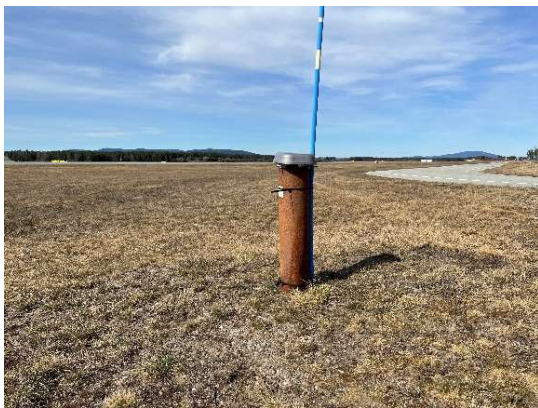
Groundwater monitoring well
