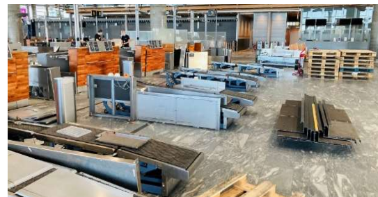
Gentle demolition for reuse options
