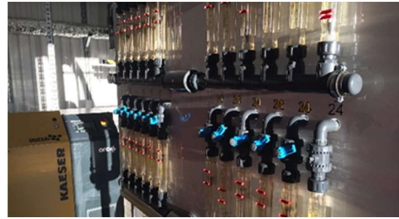
Air is pumped into the soil and groundwater to increase decomposition
