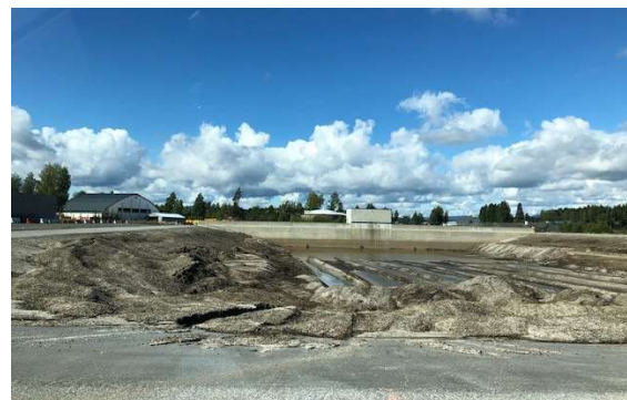
Stored snow is used for cooling the terminal in the summer
