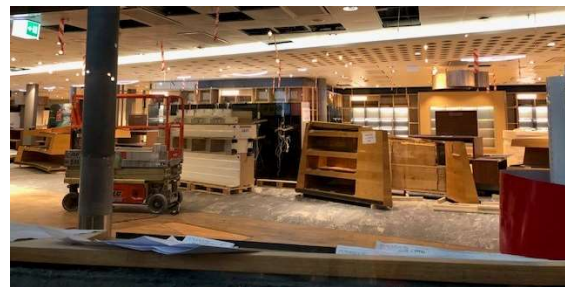
Reconstruction work in the Terminal
